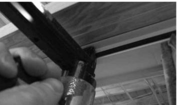
23. Install the  $3/4" \times 1-1/2" \times 1/4"$  black foam blocks to the top and bottom ends of the interlock as shown. The adhesive side of the block should face the head or sill, not the interlock.
