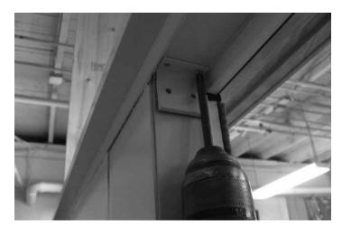
18. Install the side inactive panel stop, and fasten in place with #6 x 1-1/2" flat head screws. The stop should be justified to the top of the jamb, and should fit all the way down square in the groove in the side jamb. (It may be easier to start at the bottom of the side jamb and work your way up.)
