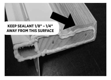
4. Apply sealant to one frame corner key. Press this corner key into place in the hollow in the side jamb cladding.
