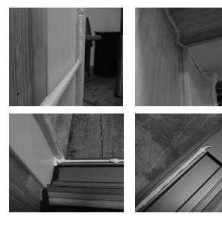
14. Using the correct panel for this side, and from the interior of the door opening - tilt the top of the panel towards you and set it onto the sill. Ensure that the sill locator on the bottom of the panel fits into the groove on the sill. The side of the panel should be all the way against the side jamb.
