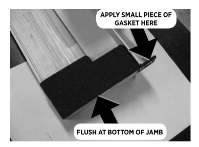
Apply sealant to the top end of the side jamb as shown below. Use caution with applying sealant near unfinished interior surfaces – if excess sealant gets smeared on interior wood surfaces, it may cause uneven finishing of wood parts after installation.
