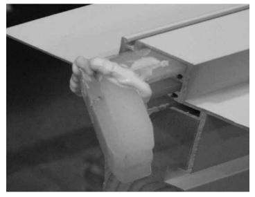
5. Align head jamb to side jamb, and push them together until the frame corner key is properly seated into both the head and side jamb cladding. Fasten the frame cladding with (2) #6 x 1-1/2" flat head screws. Seat screws evenly on opposite sides to ensure proper alignment of the corner joint – this is critical to the performance and appearance of the finished door unit.
