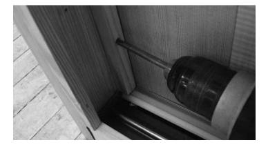
19. Install the head inactive panel stop, and fasten in place with #6 x 1-1/2" flat head screws. The stop should be justified to the side stop previously installed, and should fit all the way down square in the groove in the side jamb. 21. Install the vinyl parting bead (with weatherstrip installed) on the head, in between the inactive panel stops.
