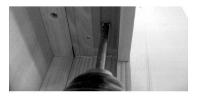
30. Install the panel bumpers to the unit by clipping the rubber profile over the rail in the sill (an alternate at the preference of the installer is to apply them to the head of the unit, fastened in place with a screw.)
